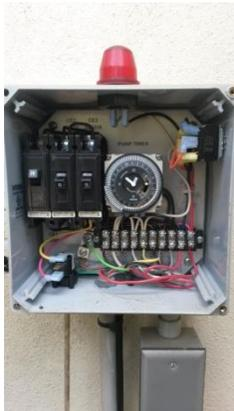
Open the box and flip any breakers that are off on.
